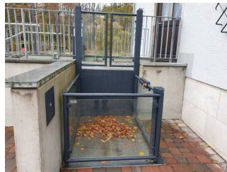
Platform lift at the entrance to the park café and park hall
